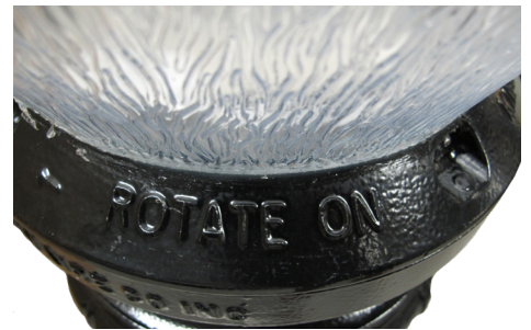
STEP 6: PLACE THE LED CONVERSION KIT GLOBE ON THE CAPITAL AND ROTOLOCK™ IT INTO PLACE OR ENGAGE THE SET SCREWS IF A NON ROTOLOCK™ GLOBE IS PROVIDED
